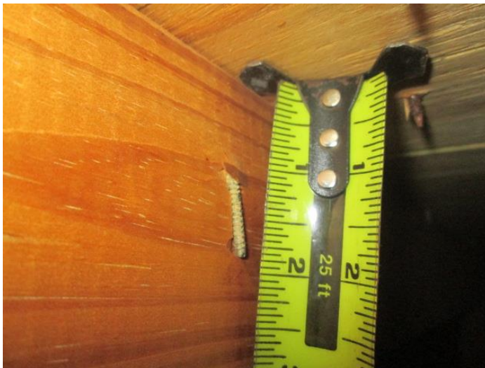
Roof Deck Attachment
