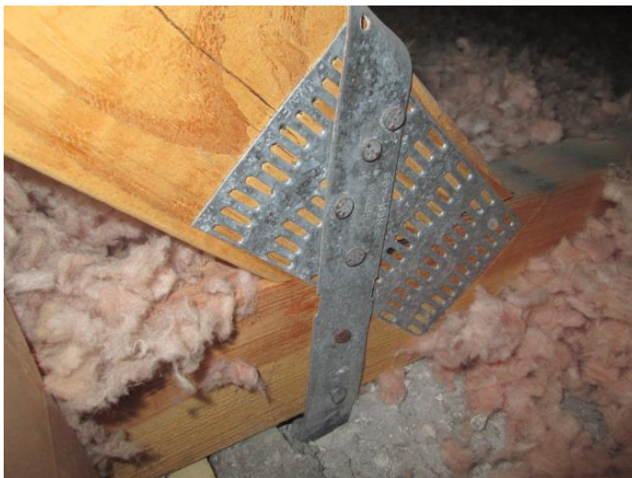
Roof to Wall Attachment
