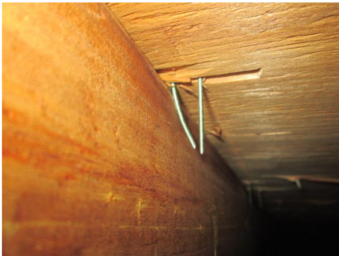
Roof Deck Attachment
