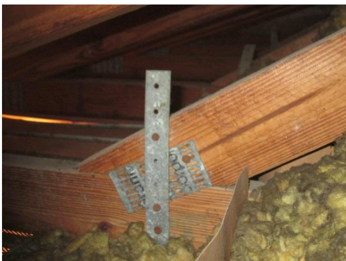
Roof to Wall Attachment
