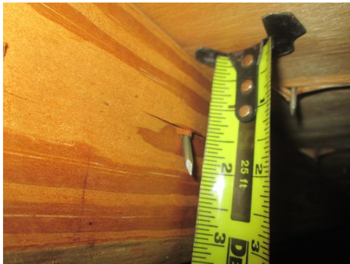
Roof Deck Attachment
