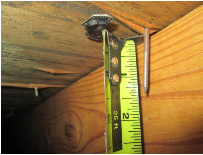
Roof Deck Attachment
