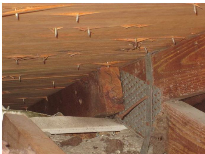
Roof to Wall Attachment
