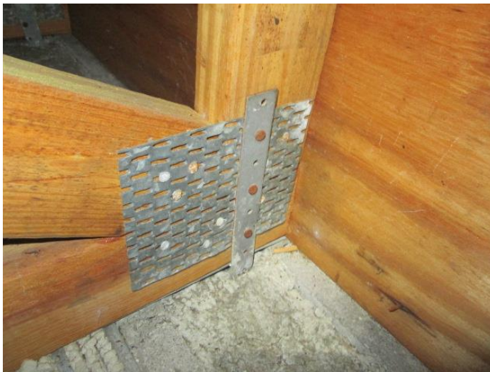
Roof to Wall Attachment
