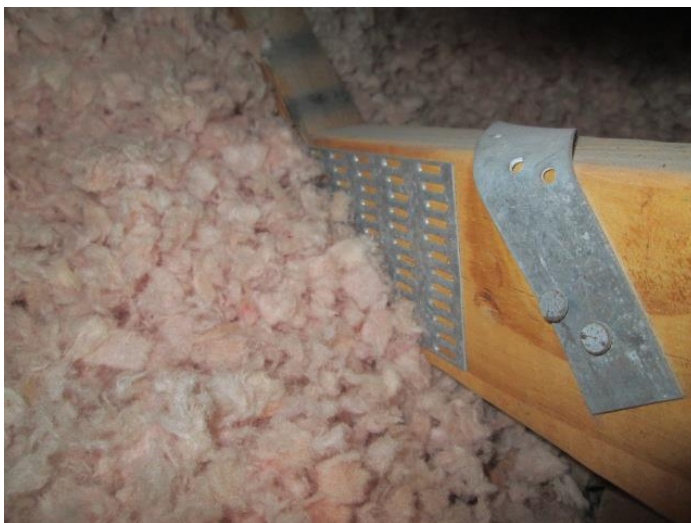
Roof to Wall Attachment
