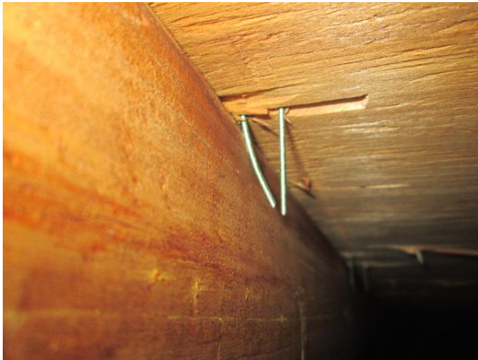
Roof Deck Attachment
