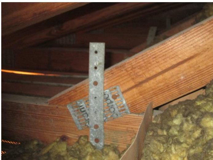
Roof to Wall Attachment
